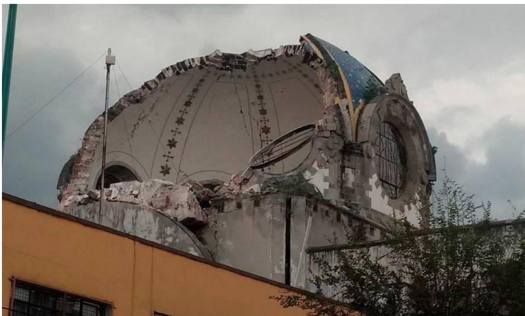
Figure 12 – Damaged dome of Catholic temple “Sanctuary of Our Lady of the Angels” as a result of the 2017 earthquake in Mexico City, Mexico.
