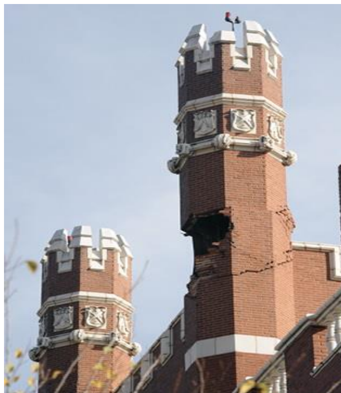
Figure 8 – Damaged Benedictine Hall turret at Saint Gregory University in Shawnee, Oklahoma USA, in the 2011 earthquake.
